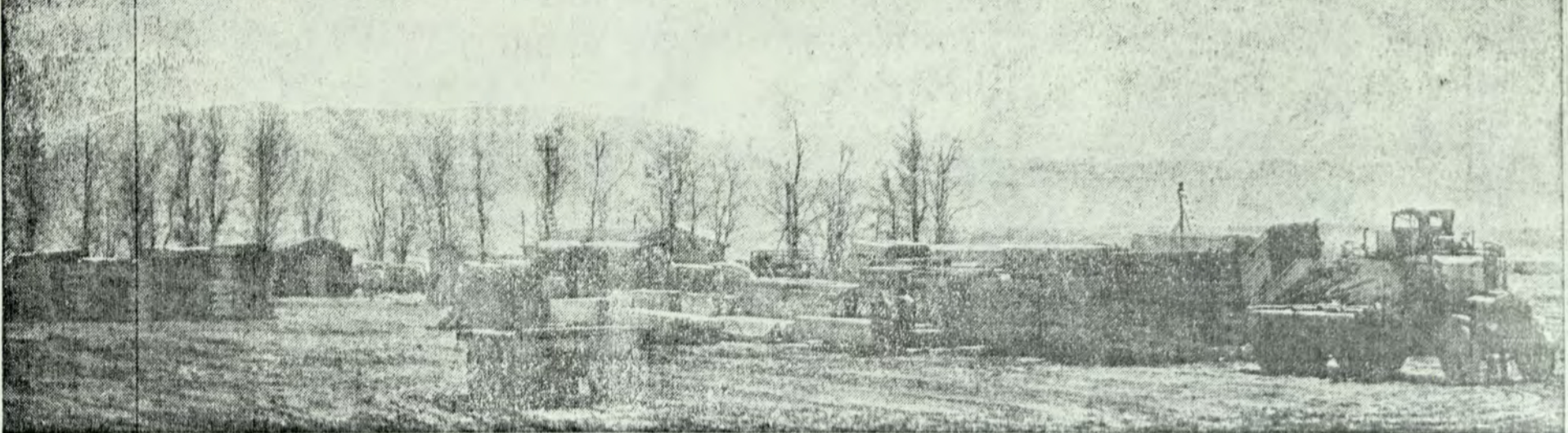
BOOM TOWN: Construction work begins on the new town for Japanese evacuees as trucks and tractors level off the ground and army of carpenters rushes building of barracks. Made simply in army style with rough boards covered with tar-paper an average of 39 barracks per day was built keeping more than 900 workmen busy.—Cut courtesy L. A. Times.
